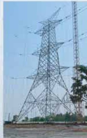
765kV D/C Tower Type 'DD/DE' Tower Test
