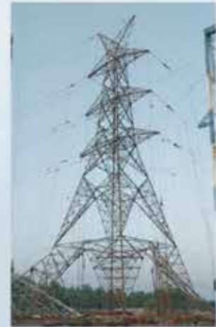
400kV D/C TT 'DBN' Tower Test
