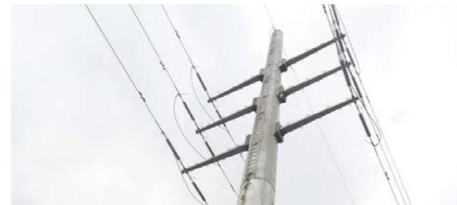
765 kV D/C - Tower
